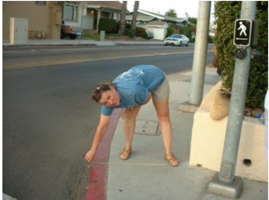
This passage around a University Avenue homeowner's wall measures just 39", well below disabled access standards.
