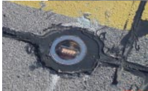
Flashing lights outline this crosswalk in San Marcos to alert drivers when pedestrians are crossing the street.
