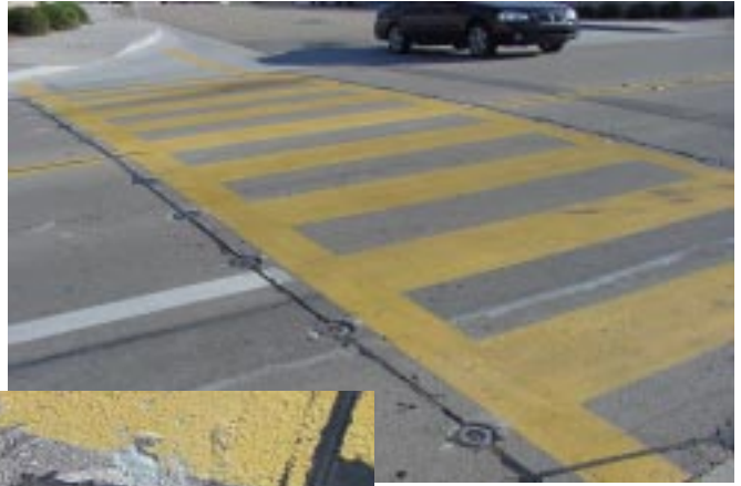
Flashing lights outline this crosswalk in San Marcos to alert drivers when pedestrians are crossing the street.
