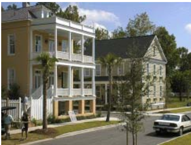
“New Urbanist” developments feature narrow, walkable streets — and achieve 20% higher resale value.
