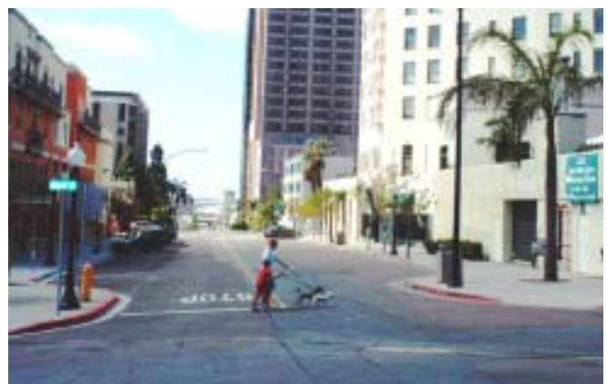
Curb extensions at this downtown San Diego intersection make it "Family Safe".
