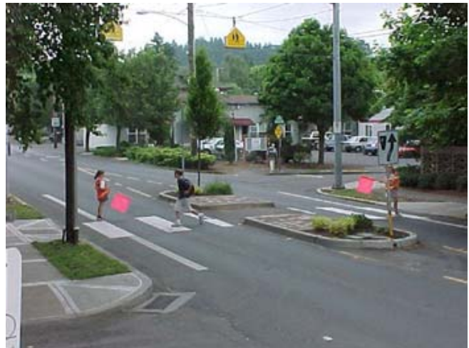
A raised refuge island and crosswalk similar to this one is being planned for Adams Avenue.
