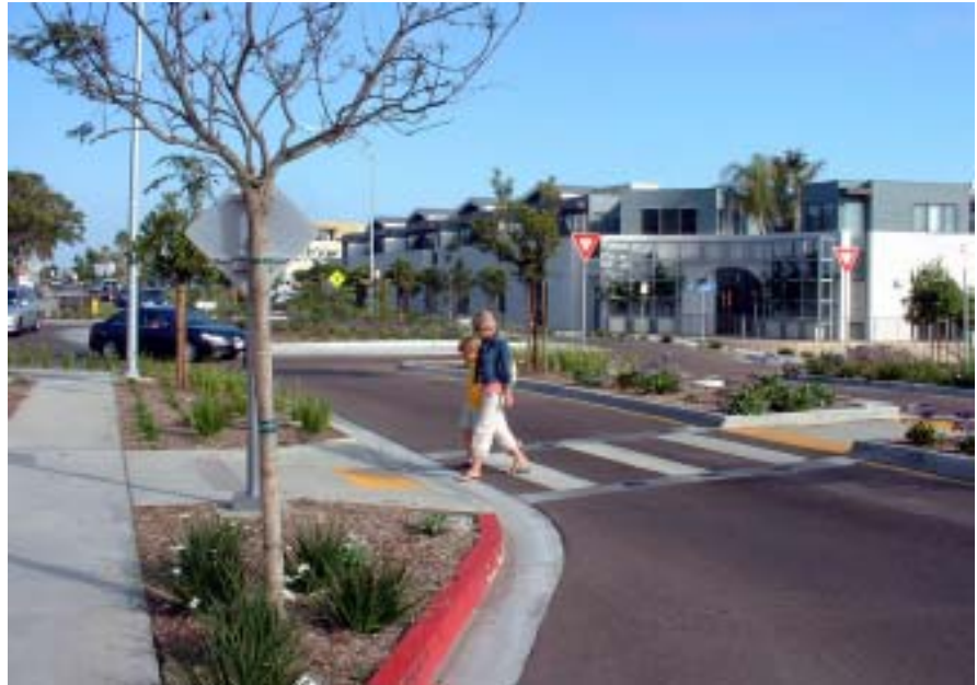
Traffic-calmed La Jolla Boulevard allows drivers, bicyclists, and pedestrians to safely share the street.
