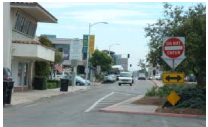
The channelization island at Washington Place should be altered to serve as a traffic calming device.
