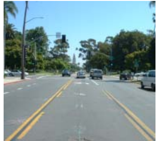
Laurel Street at 6th Avenue – the only controlled crossing point for pedestrians accessing Balboa Park from 6th Avenue.
