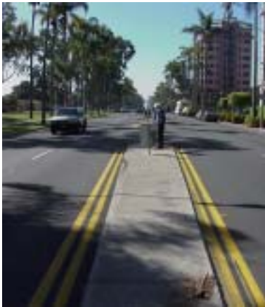
Narrow medians function as de facto pedestrian refuges. With fewer lanes, expanded refuges could be accommodated.
