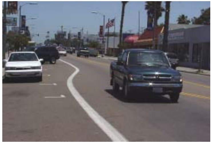
Diagonal parking creates a lane shift – a form of “chicane” that induces slowing.
